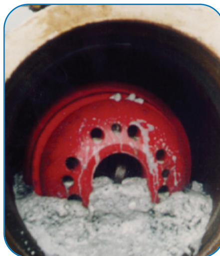
Gas Hydrates from a subsea flowline
